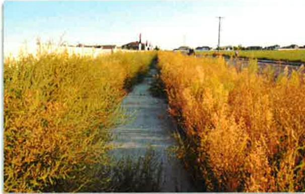
*Example of a poorly maintained sidewalk near the Prairie Breeze housing development on the west side of Five Mile Road. Where there are no adjacent landowners to shovel sidewalks and mow swales, it is especially important that they be constructed in a manner to minimize maintenance requirements.*
